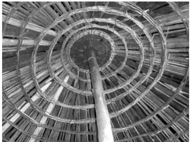
Figure 4 Central pole in a circular house, Omo Valley, Ethiopia.
